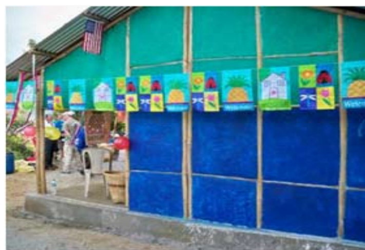
Completed Habitat home in Pokhara, Nepal.
