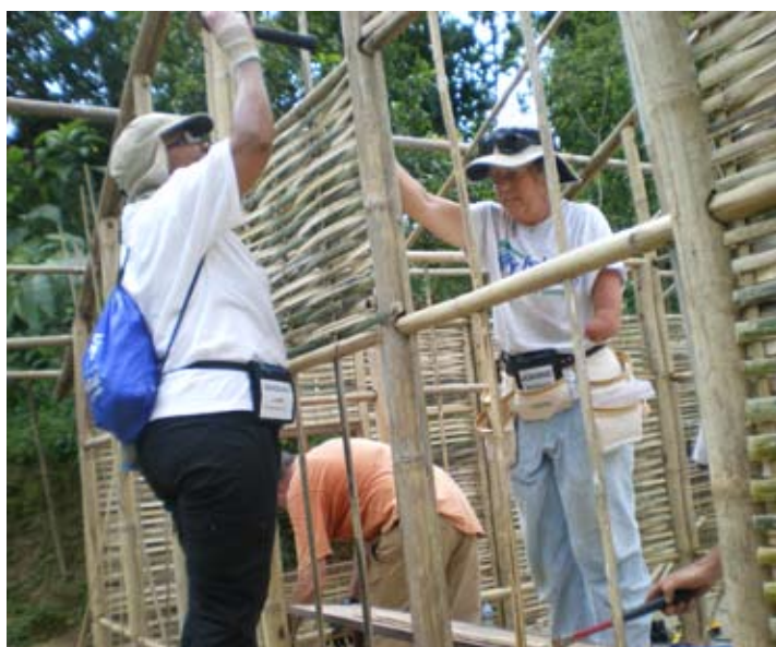
Joanne works on bamboo walls.
