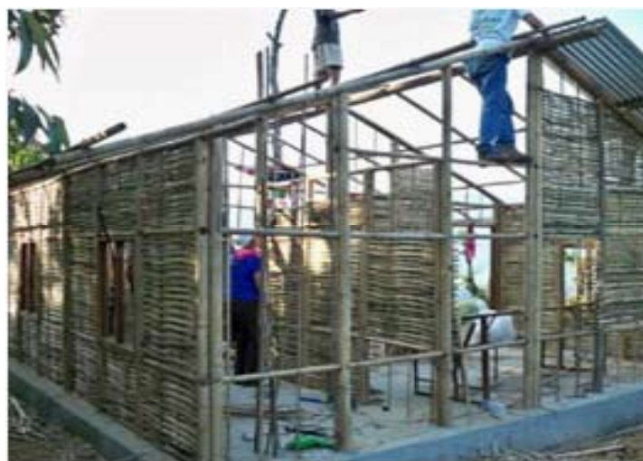
Walls are woven with bamboo strips.
