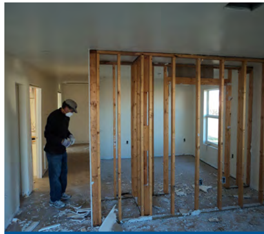
Chinese Drywall is Remediated
